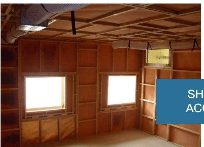
CHS, in partnership with Simon Hegele and shielding manufacturer Tekemi, provide RF Shielding systems that are primarily constructed of wood backing and copper sheeting.
